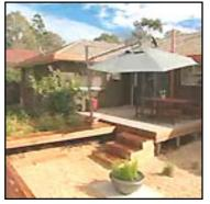
The cantilevered boardwalk was constructed from 90x90mm treated pine posts, 140x140mm treated pine bearers and 90x45 joists. Merbau hardwood decking was laid.
